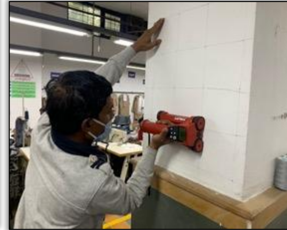
Structural Safety: Ferro-Scanning Test
