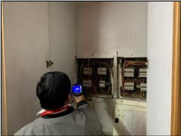
Electrical Safety: Thermo-graphic Test
