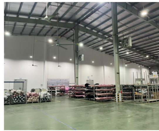
Fire-rated wall and doors built between the warehouse and production area.
