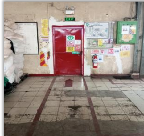
Emergency Pathway Secured
