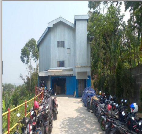
No Emergency Exit Observed
