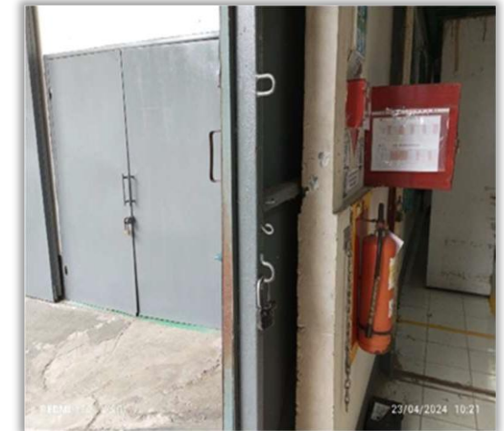
Locking mechanism on exit door
