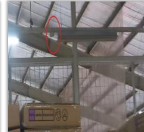
Local Type Smoke Detector Observed
