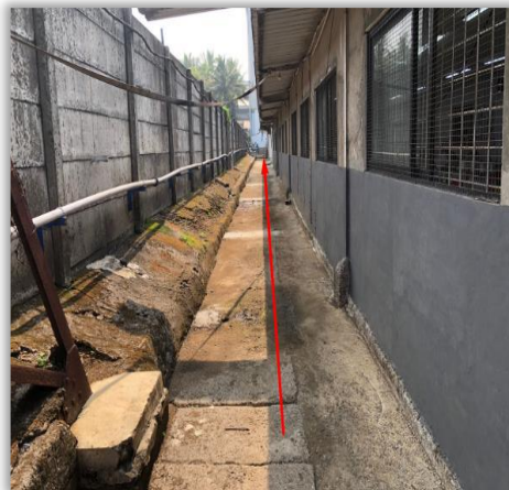
Additional Exit Provided
