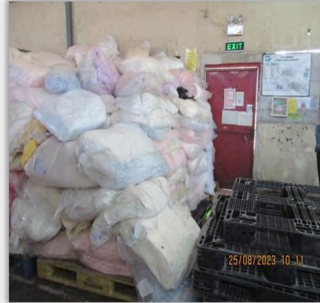
Obstructed Emergency Exit
