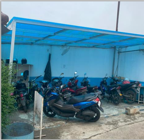
Broken Roofing Replaced
