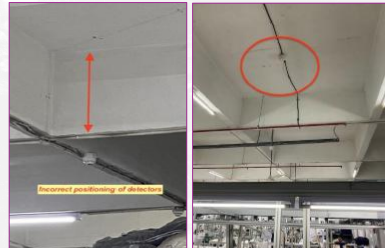
Smoke detector positioning before and after
