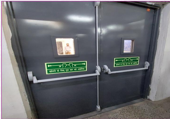
Push bar has been install over doors
