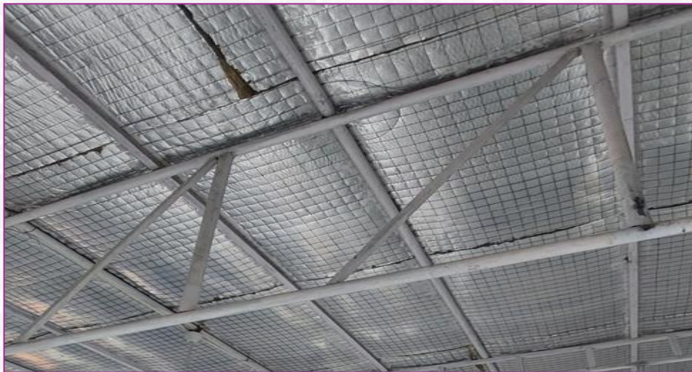
Bracing to MS structure
