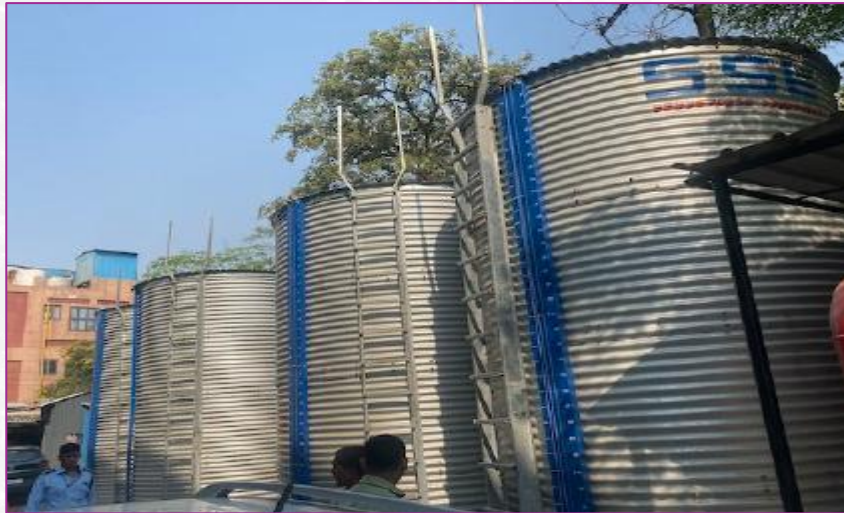
Additional water tanks installed by factory
