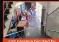
Exit passage blocked by vending counter
