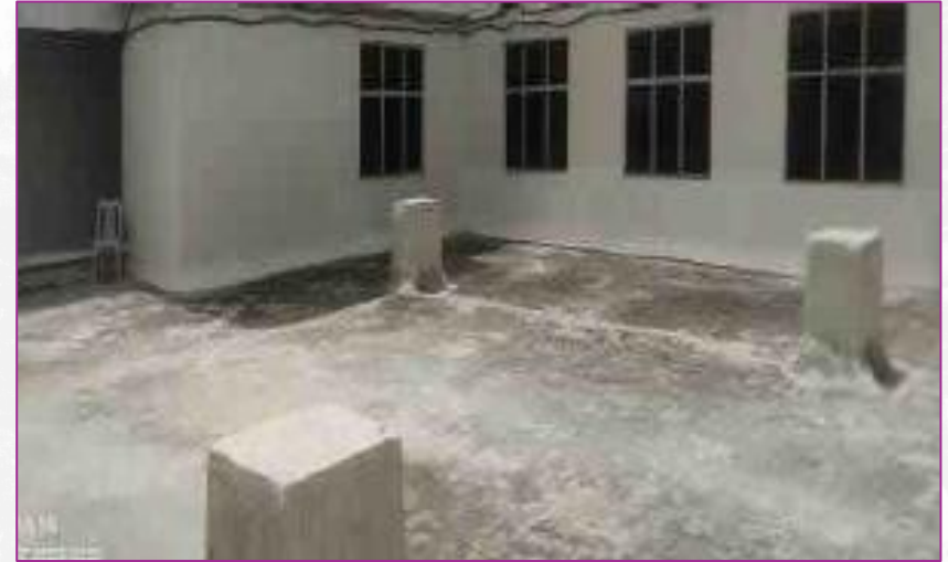
Corroded bars were repaired from column
