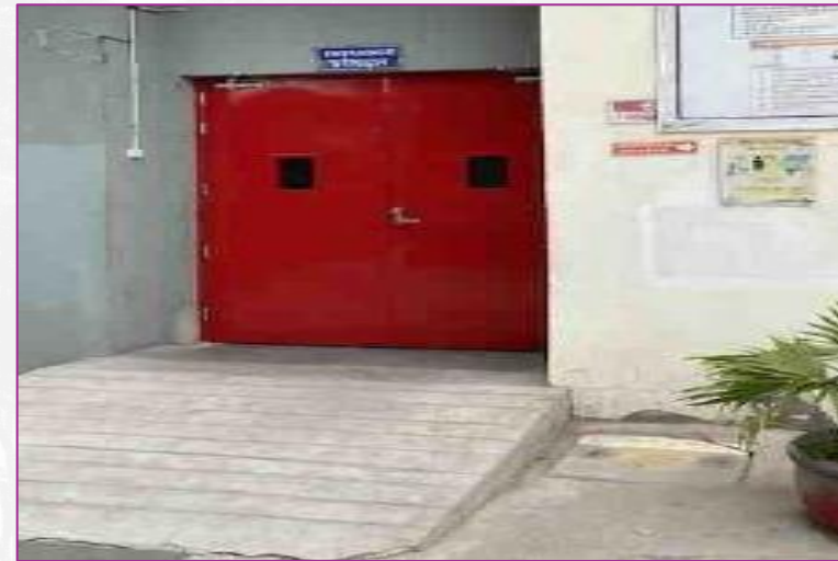
Fire door has been installed
