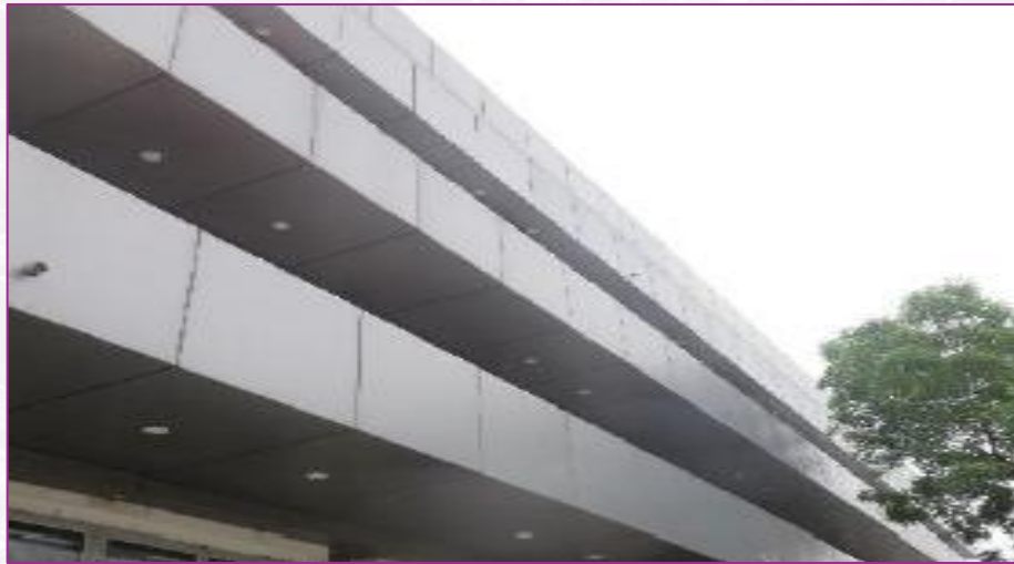
Corroded structure repaired and covered
