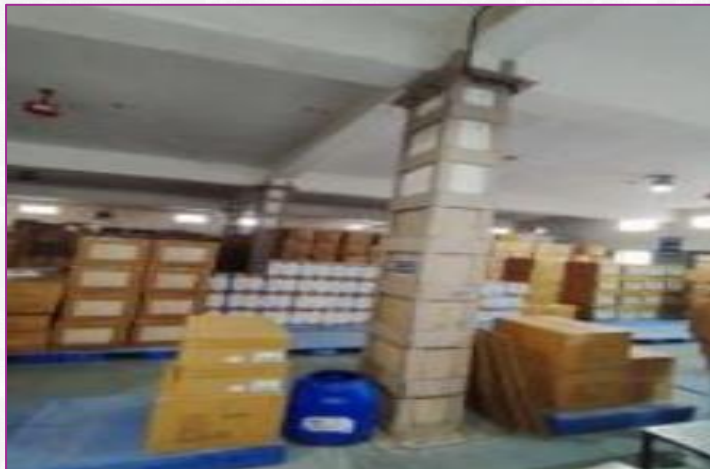
Jacketing provided for column level below
