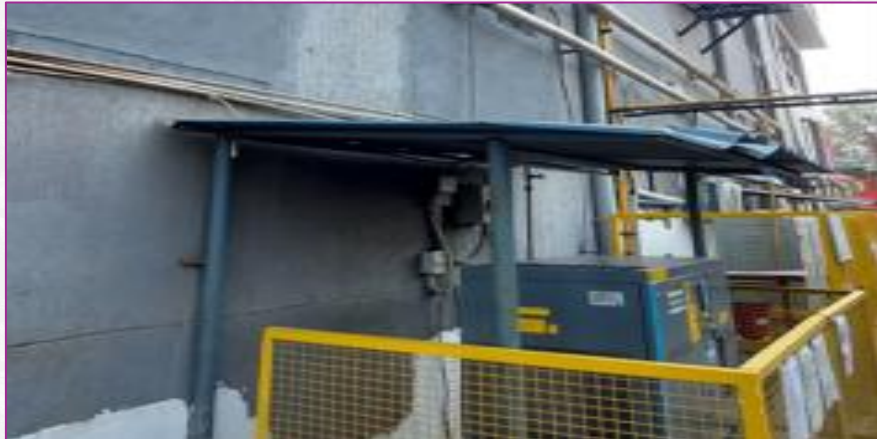
Window opening towards compressors has been closed
