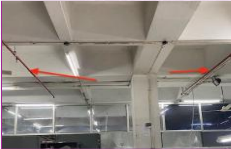
Additional water tanks installed by factory
