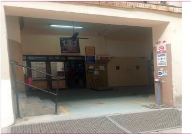
Rolling shutter has been removed
