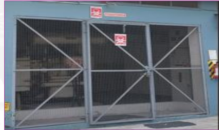
Warning signage provided
