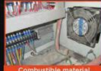
Combustible material inside electrical panel
