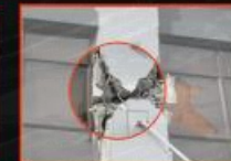
Crack in the pillar
