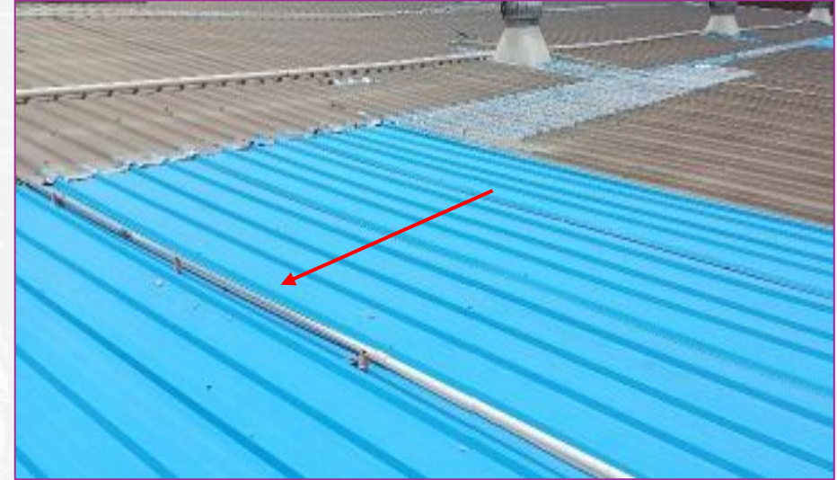
Eearthing provided to MS truss
