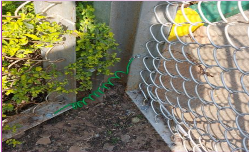
Bonding provided over transformer gate
