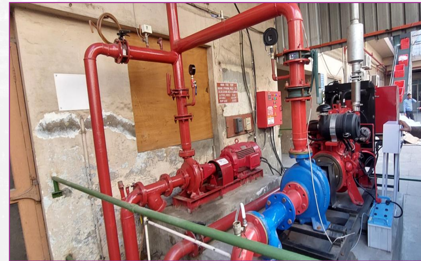
Backup Fire pumps are installed
