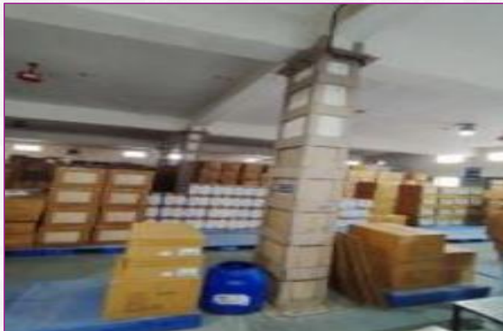
Jacketing provided for column level below
