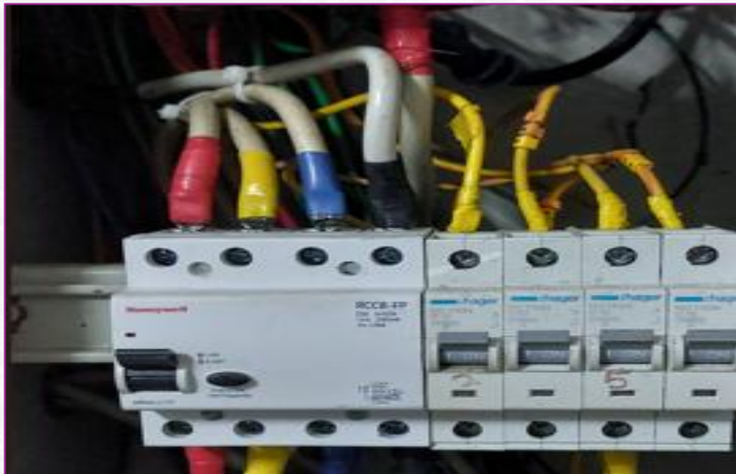
Lugs provided for electrical panel
