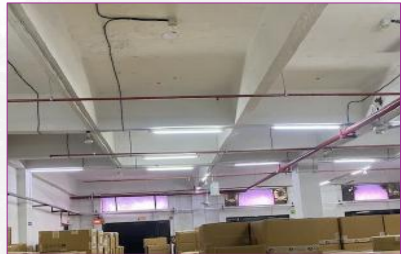
Sprinklers installed in material store
