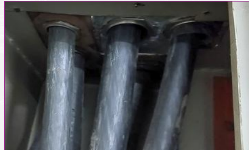
Glands provided over electrical panel
