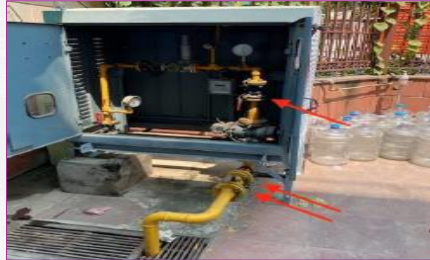
Bonding provided over LPG gas pipeline
