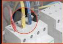
Lint/dirt on electrical panel
