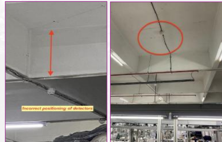
Smoke detector positioning before and after
