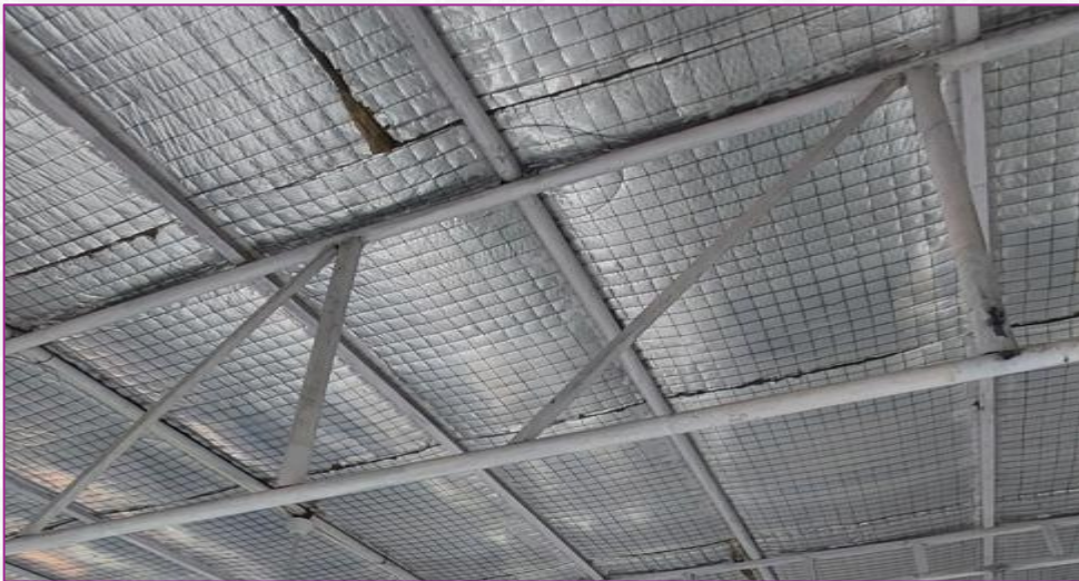
Bracing to MS structure
