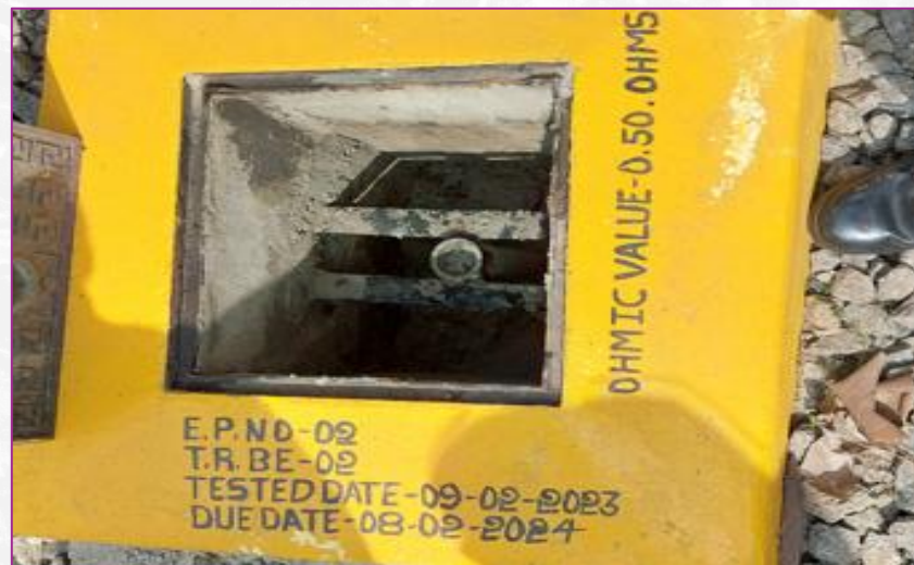
Earth pit maintained and monitored
