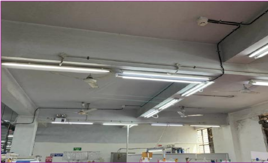
Smoke detector installed
