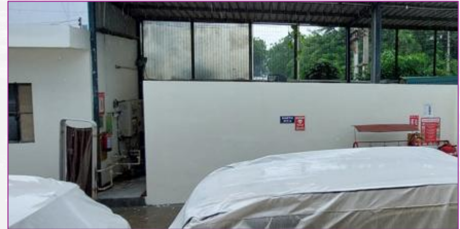
Wall separation provided between transformer & evacuation route
