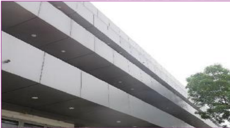
Corroded structure repaired and covered
