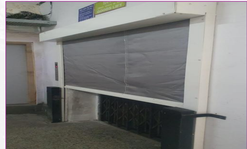
Panel room enclosure by fire door
