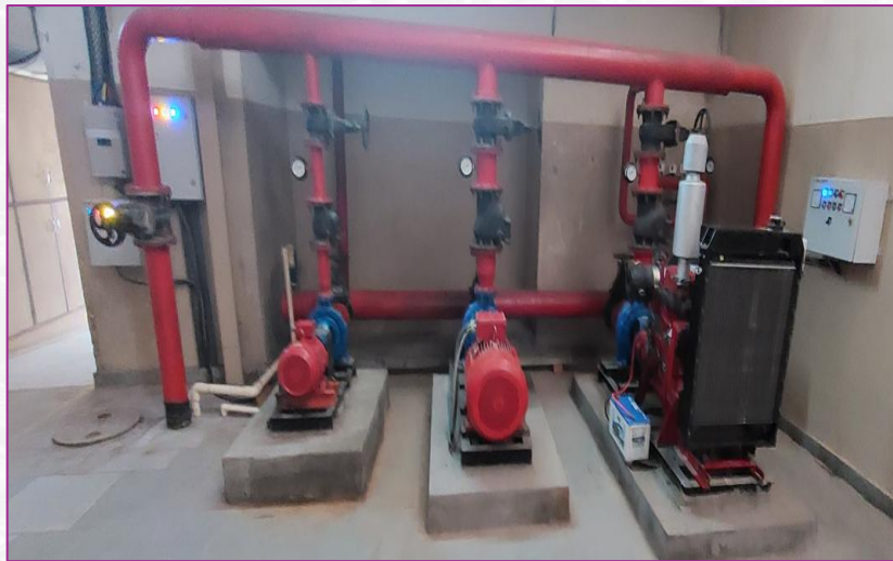
All 3 Fire pumps are installed
