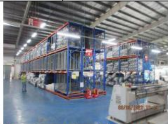
Figure: Storage and production area was stocked beside production area of factory 1, no fire separation
