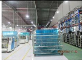
Figure: Fabric storage and production area was stock beside production area of factory 8, no fire separation
