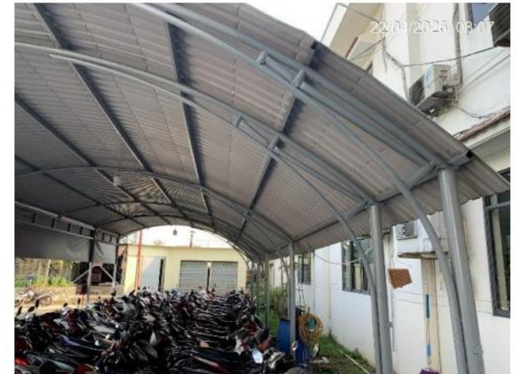
Figure: Retrofit for roof frames of the parking.
