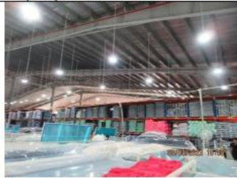
Figure: Storage and production area was stock beside production area of factory 2 , no fire separation
