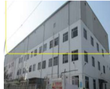
LPS system not installed in factory
