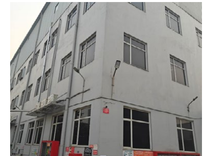
Dampness has been repaired
